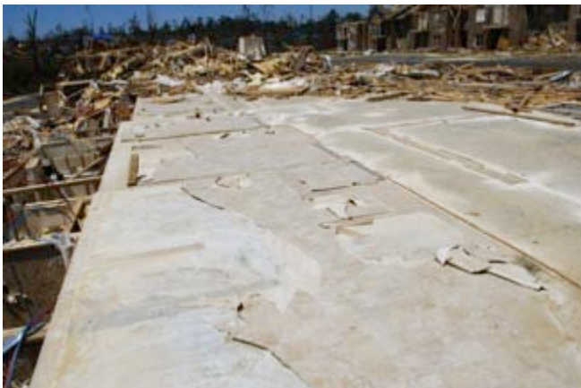
Figure 5.13 Slab swept clean in newer 2010 construction
