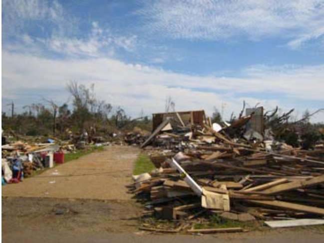
Figure 5.12 Most walls collapsed
