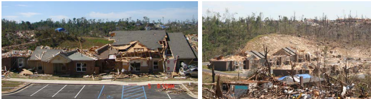
Figure 4.8: Badly damaged and partially destroyed apartment complex
