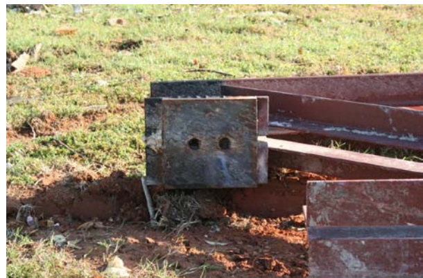
Figure 4.16: Roof truss that was lifted off during tornado; diagonal member buckled (not shown here).
