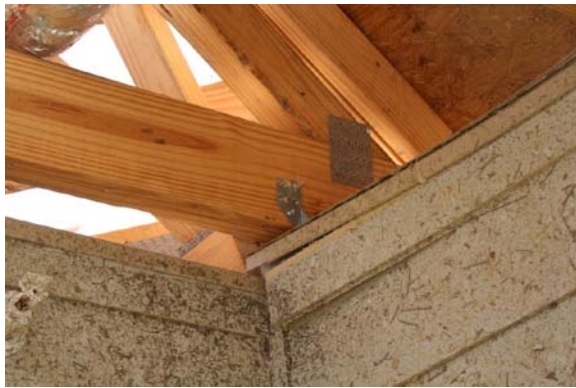
Figure 4.9 Photograph of installed hurricane clip
