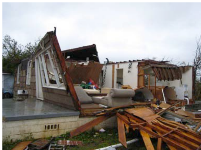
Figure 5.11 Exterior walls collapse
