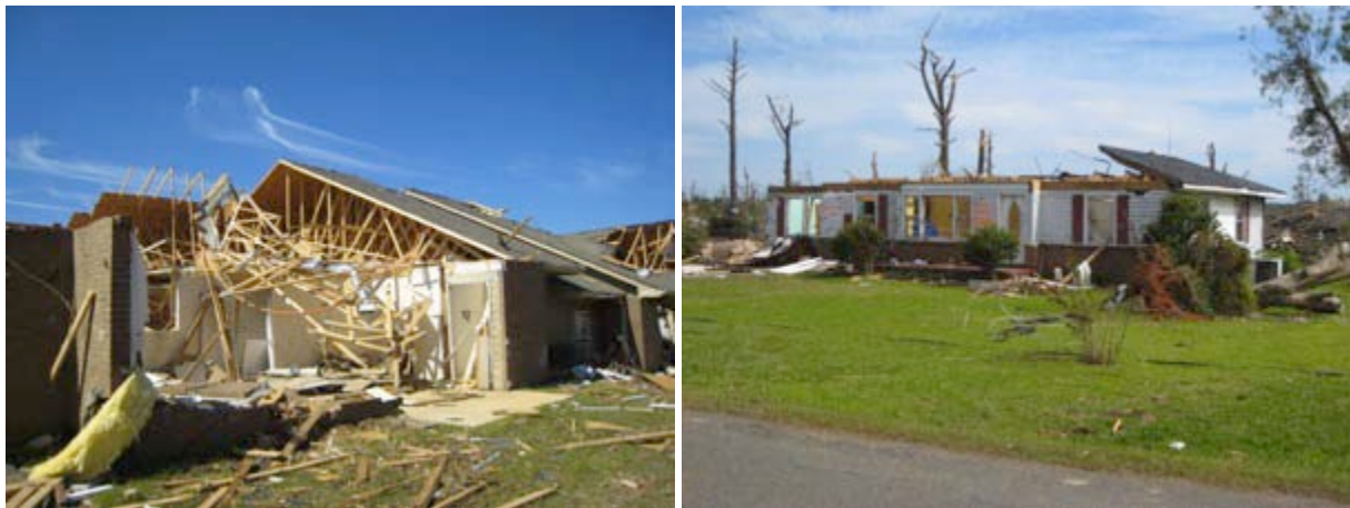
Figure 5.10 Large sections of roof removed
