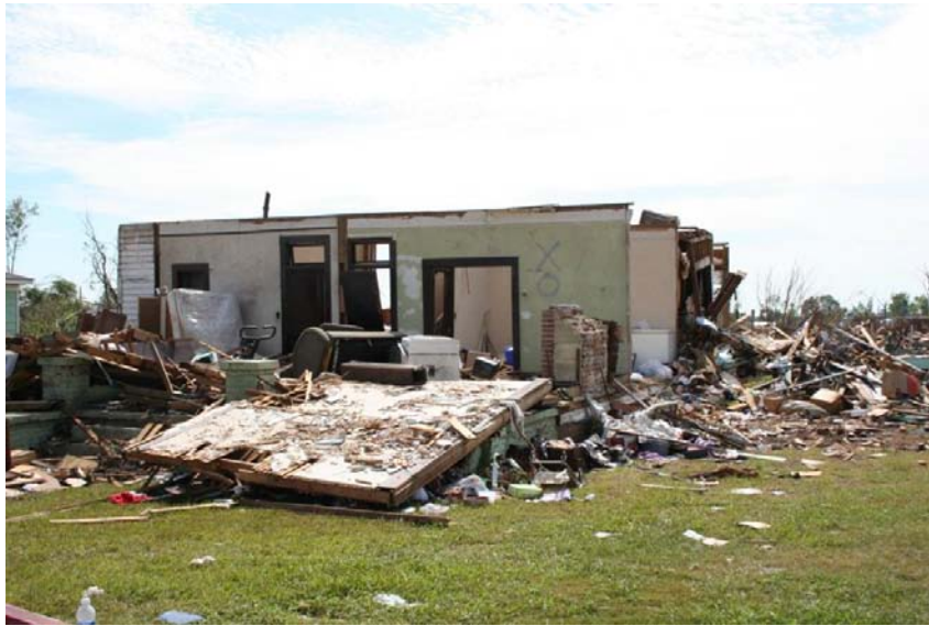
Figure 4.5 Interior walls collapsed
