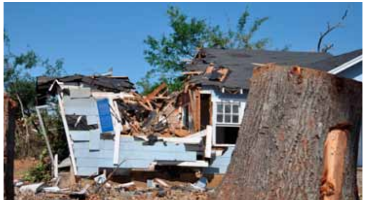
Figure 2: Tree fall caused severe building damage.
