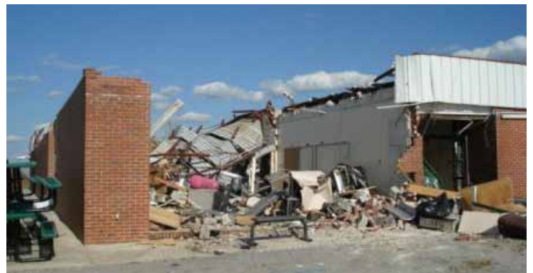
Figure 4: School Buildings, Hackleburg, AL
