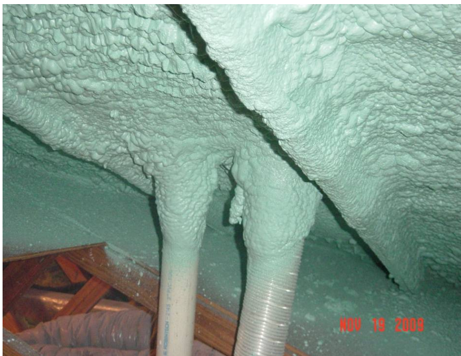
Figure 3.2: ccSPF sprayed to seal openings where hose/pipes pass through the roof deck
