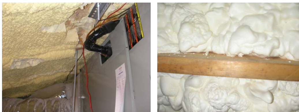
Figure 3.3: House 1 with ocSPF installed in the attic
