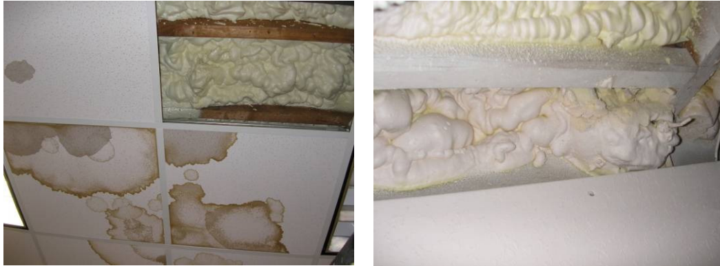
Figure 3.4: Office roof with ocSPF installed
