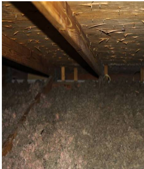
Figure 5.10: Blown Insulation and protruding nails from sheathing
