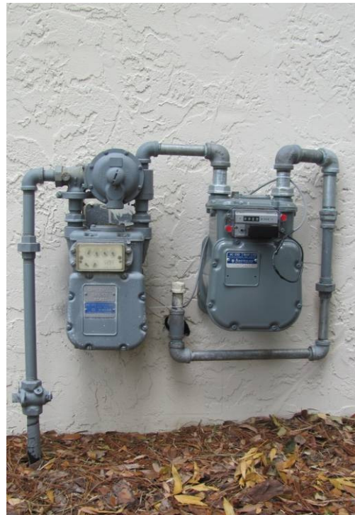
Figure 8.8: Gas Meter with digital pulsar (right) placed in parallel with existing meter (left)
