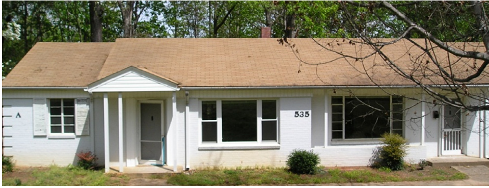
Fig. 1. Douthit Hills duplex residential structure.
