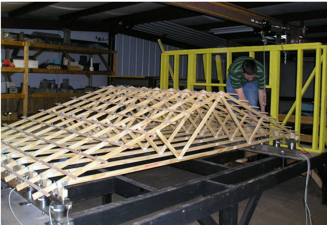
Figure 2.7 – Completed 1:3 scale model roof
